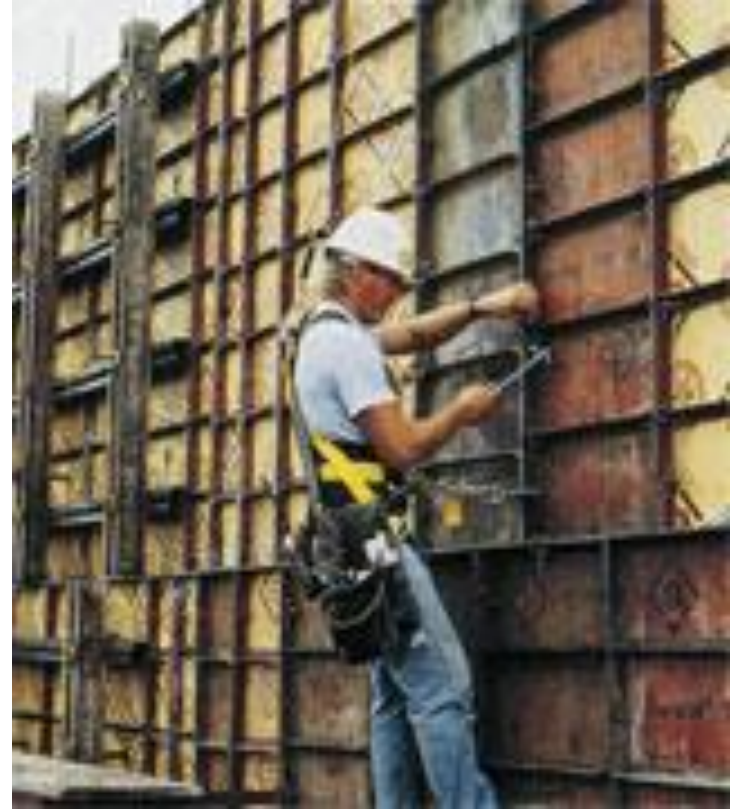
WALL FORM WORK
