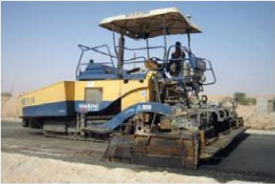
Finisher (Asfalt Serme)
