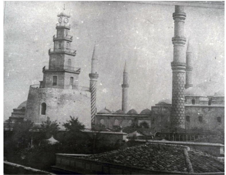
The timber structure between 1884-1894 (Archives of Edirne Museum)
