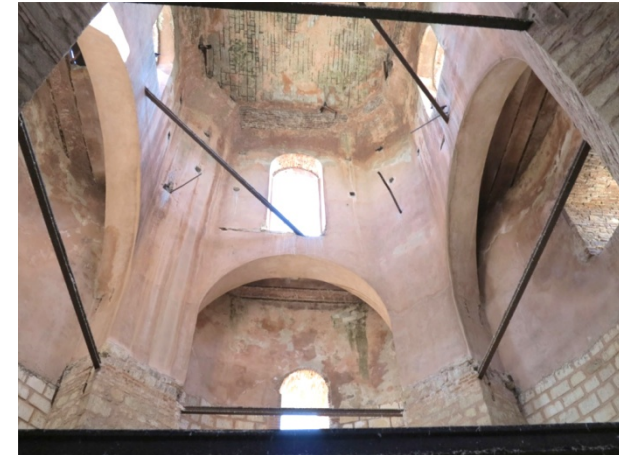
Reinforced concrete roof of the tower (2014)
