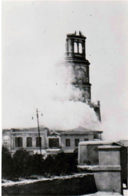
The masonry structure, 1953 (Archives of Edirne Museum)
