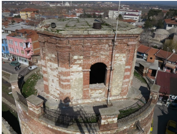
The roof of the tower
